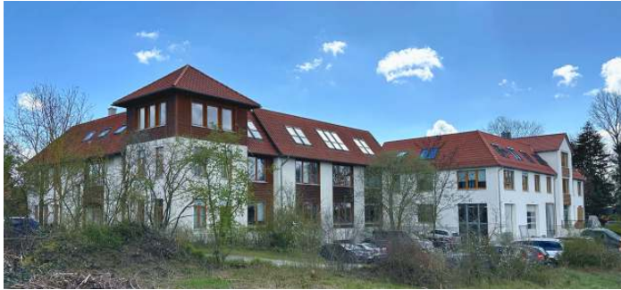
Development Department, Kolshorner Straße
