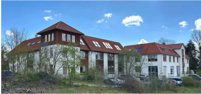
Development Department, Kolshorner Straße
