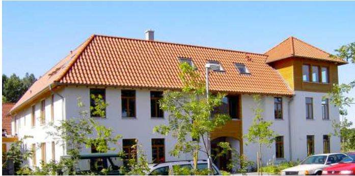
Development Department, Kolshorner Straße
