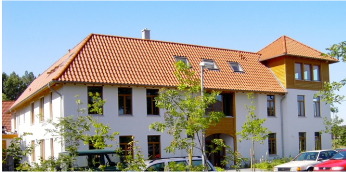
Development Department, Kolshorner Straße
